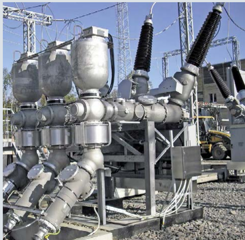
Fig. 20: 3AP1 DTC 145 kV with voltage transformer and cable connection
